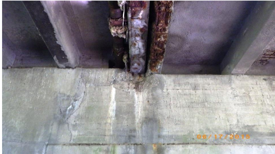
Figure 5: Example of Concrete Deterioration on a Municipal-Owned Bridge
