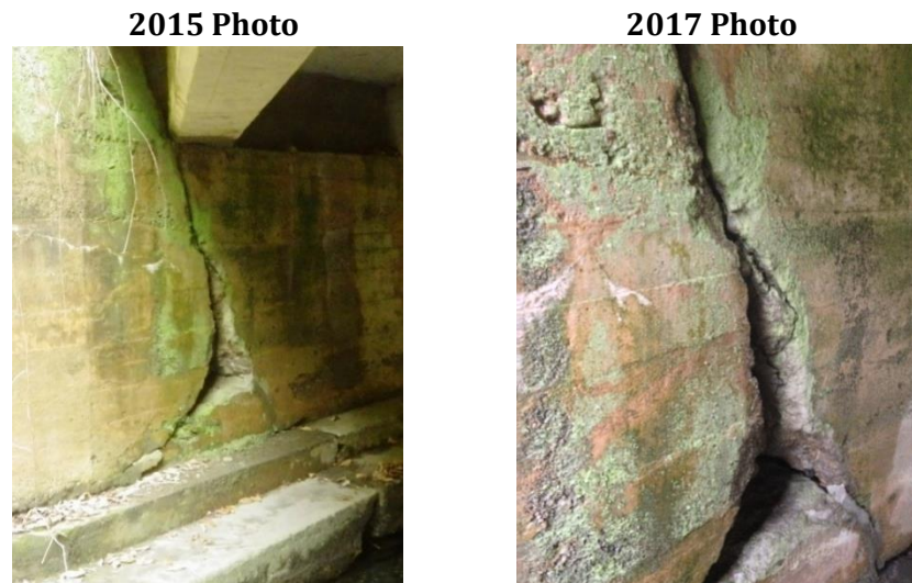
Figure 8: Crack in Randolph Bridge #36 Abutment
